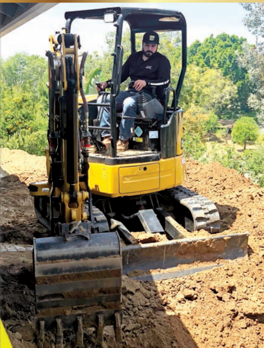
Left: Lux Landscape Design's Cat 303E CR mini excavator performs a difficult cliffside pool excavation in Fallbrook.
