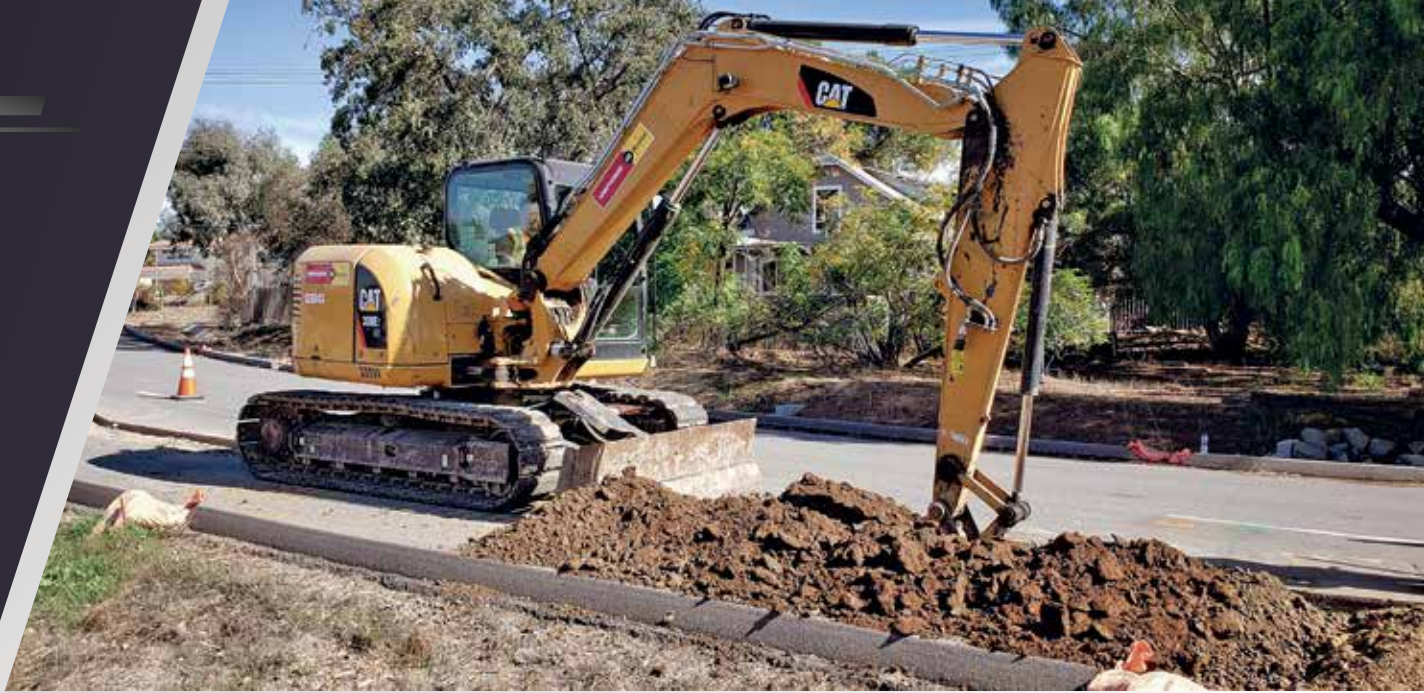
Above: LB Civil Construction rented a Cat 308E2 CR excavator from Hawthorne Rentals for a trench excavation project for Valley Center Municipal Water District.
