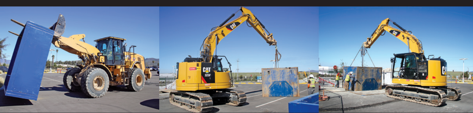
Above: ACCO using Cat 950M wheel loader and Cat 325F excavator rented from Hawthorne Rentals to move and place trench box on warehouse distribution project.
