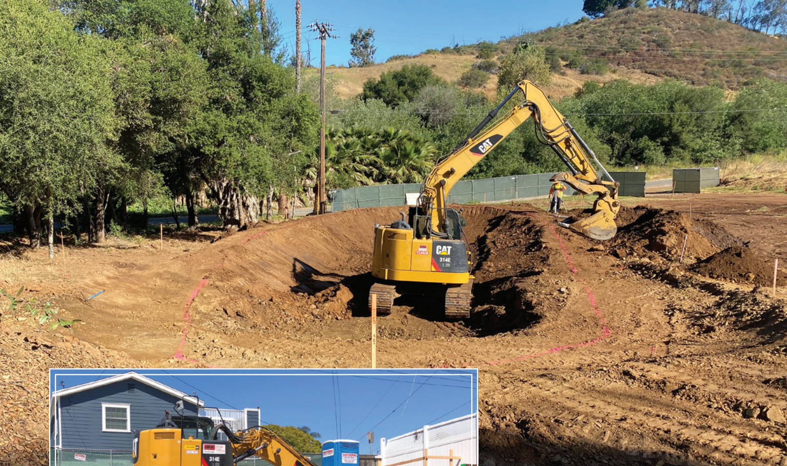
Above: Installation of biofiltration basin and drains in San Marcos.
