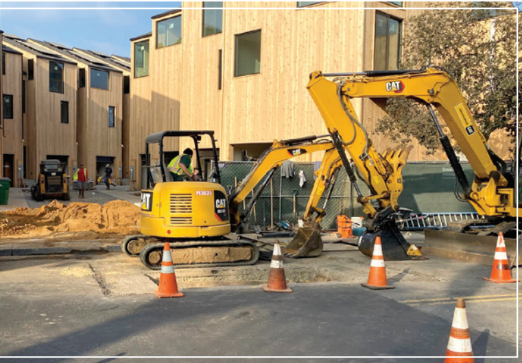
Left & Above: MB General Engineering, Inc. performing a tie-in from a private PVC storm drain to public RCP storm drain in Carlsbad.
