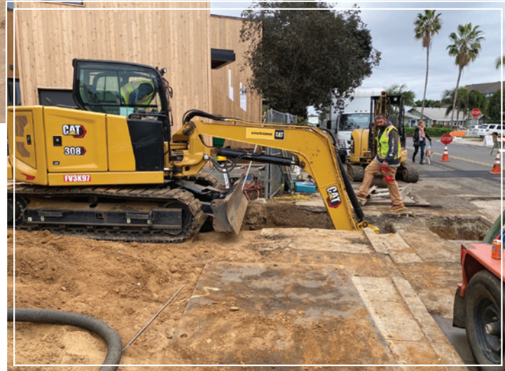
Left & Above: MB General Engineering, Inc. performing a tie-in from a private PVC storm drain to public RCP storm drain in Carlsbad.
