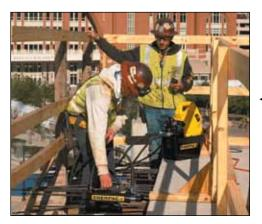
■ Designed to be tough, the ZU4-Series with steel reservoirs will take the abuse of today's construction sites. The ZU4908JE is the ideal pump for post tensioning applications. For post tensioning tools see page 180.
