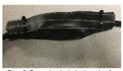
Step 3: Securely zip tie both ends of the protective sleeve.
